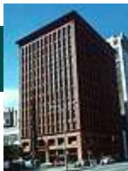
Sullivan and Adler: Guaranty Building, Buffalo, 1894-95
