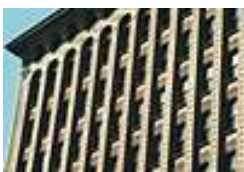
Sullivan and Adler: Guaranty Building, Buffalo, 1894-95
