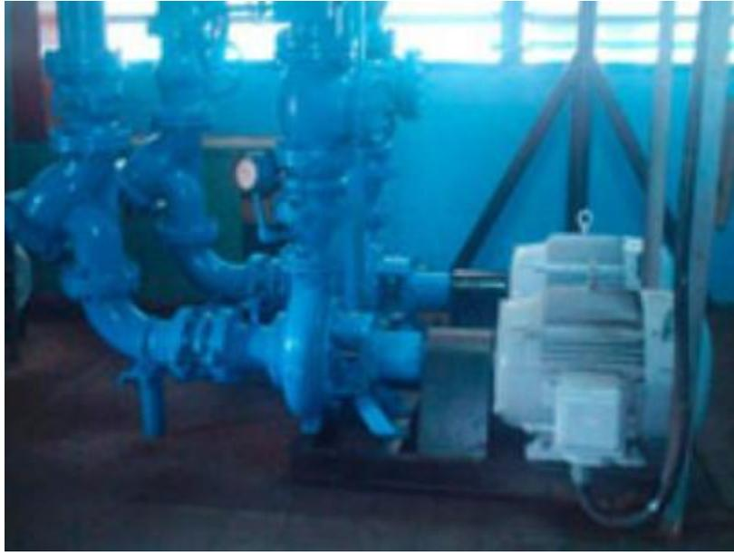
(Gambar 4. Chilled Water dan Condenser Water Pump)
