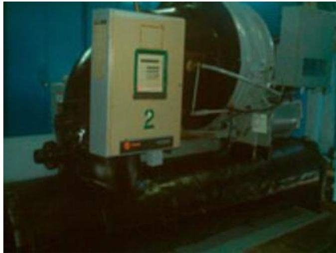
(Gambar 2. Water Cooled Centrifugal Chiller)
