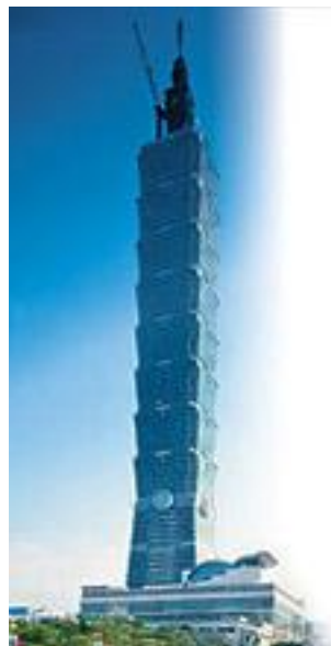
Eight-floor modules with outward leaning facades emerge from lower 26 floors. (Photo courtesy of Joseph Gartner & Co.)
