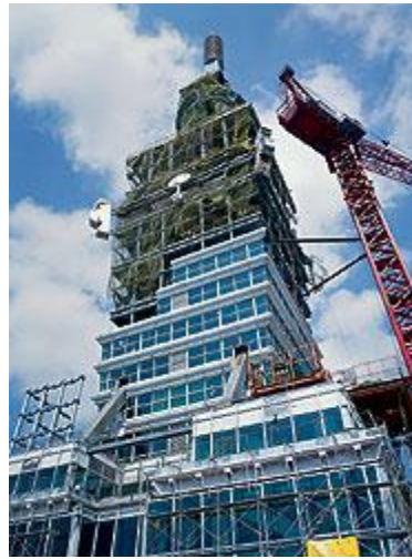
Curtain wall installation almost complete. (Photo courtesy of Joseph Gartner & Co.)
